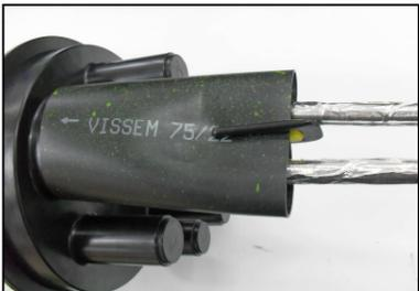
When using dual type heat shrink tube, insert the split clip as the figure shown before heating the tube
