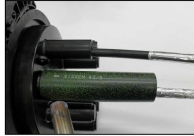
Push the heat shrink tube up to the cable inlet port end, and heat the tube starting at the inlet port moving away from it while controlling the fire.
